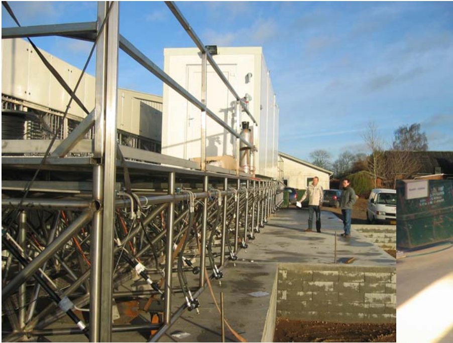
Left: Main structure before it was transported to sea
